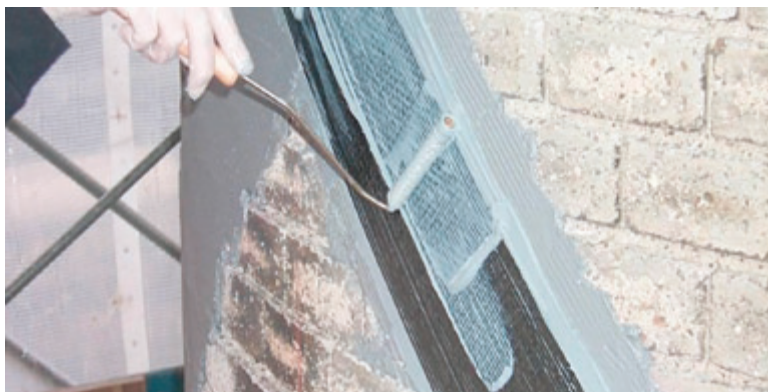
Figure II-5 : Application du SikaWrap® :[15]
